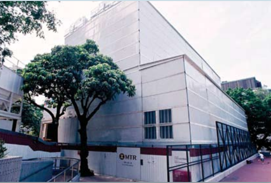
佐治五世紀念公園的隔音罩已經建成，爆破工程將於七月進行。 Noise enclosure at the King George V Memorial Park is completed and blasting works are anticipated to commence in July.
